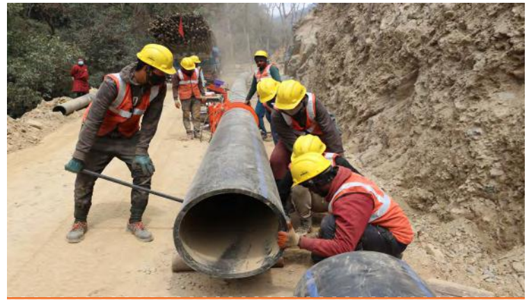
Workers in Bhutan address Phangyul's water scarcity with the installation of a pressurized piped irrigation scheme, retrofitted with new and climate-resilient technology. The new irrigation will benefit 24 villages and more than 1,300 acres of agricultural land.
