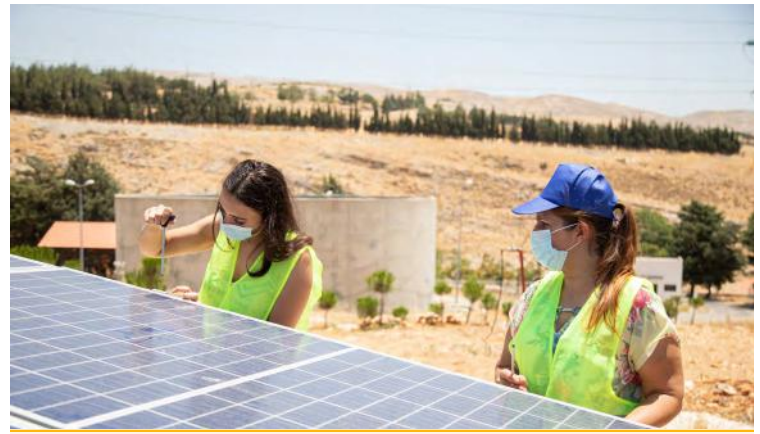
In Lebanon, women install solar panels as part of efforts to empower women in the renewable energy sector, improving their skills for economic empowerment during crises and the pandemic.
